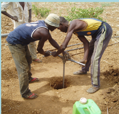
Manual drilling operation using auger technique in Niger. ©Kerstin Danert
