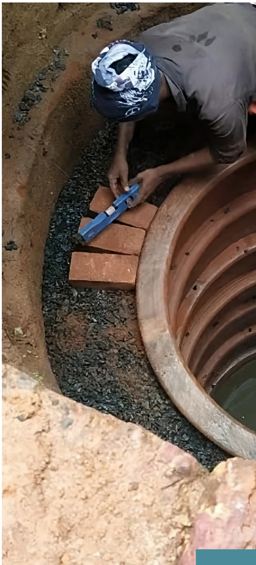
Water well lined with clay rings in India. ©KK Clay Works
