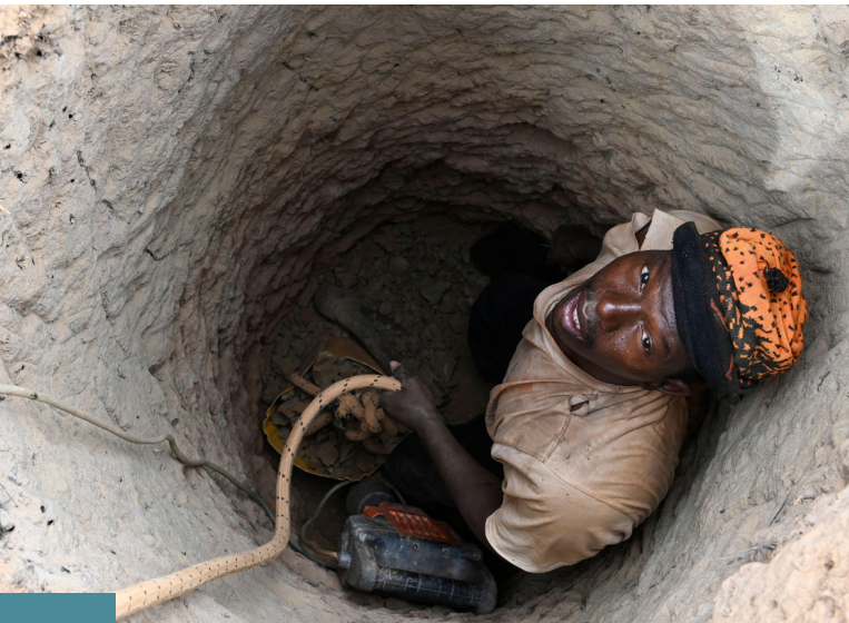
Well digging with a Jackhammer, Mali. @Joerg Boethling / Alamy Stock Photo
