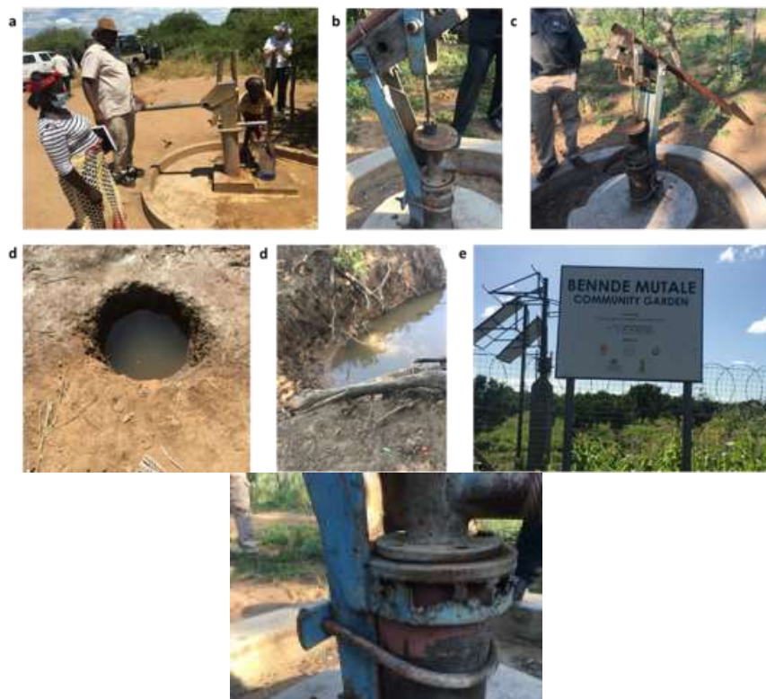
Figure 25: Borehole types and groundwater use (a) Afridev hand pump used for community water supply in Mozambique (b) Zimbabwe Bush hand pump (c) dysfunctional hand pump in the vicinity of Malipati village (d) unprotected well used for domestic water supply in Mozambique (e) unprotected abstraction directly from the Limpopo River in Mozambique
