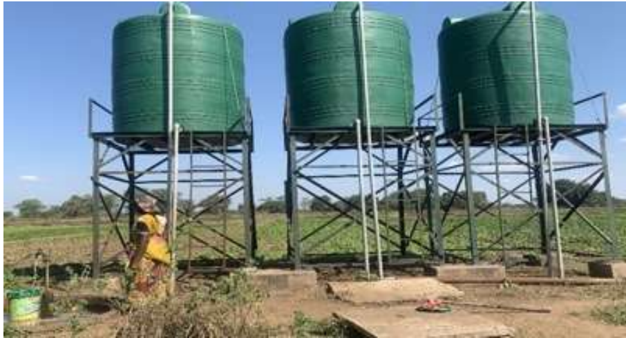
Figure 6: Women-run Irrigation system in the Sengwe Communal Area, Zimbabwe.
